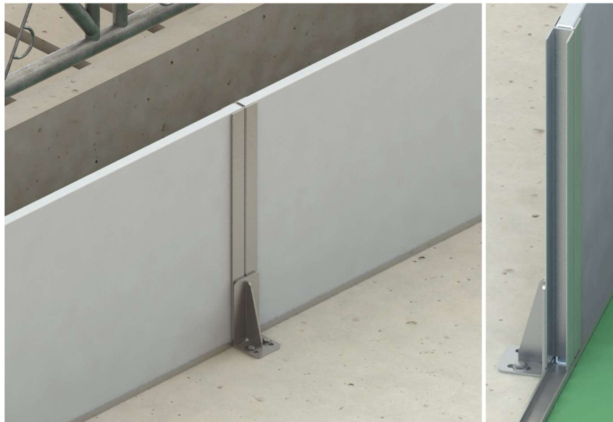
Fig. 13 Modular wall system installed
