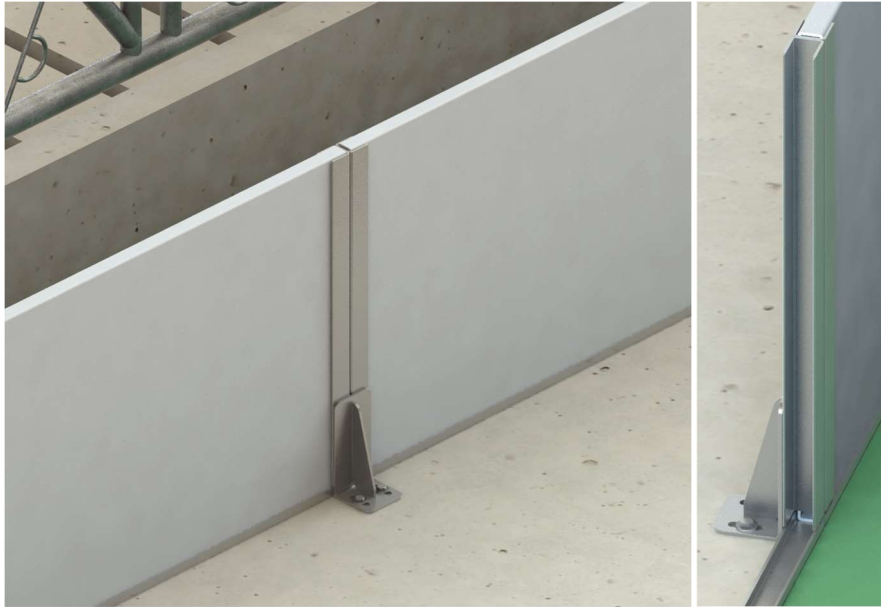
Fig. 13 Modular wall system installed
